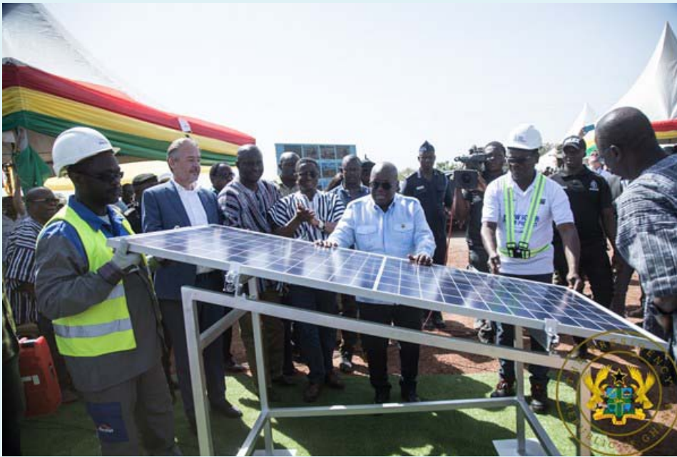
The President, being assisted by VRA's Projects Manager, Mr. Isaac Bedu, to cut the sod
